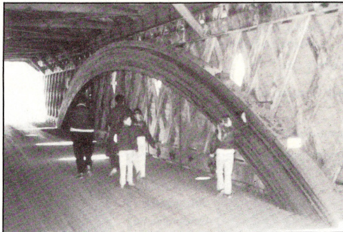
The laminated arches in the restored bridge were made of 22 2x12x20-foot pine timbers which came from Cotton Hanton.
